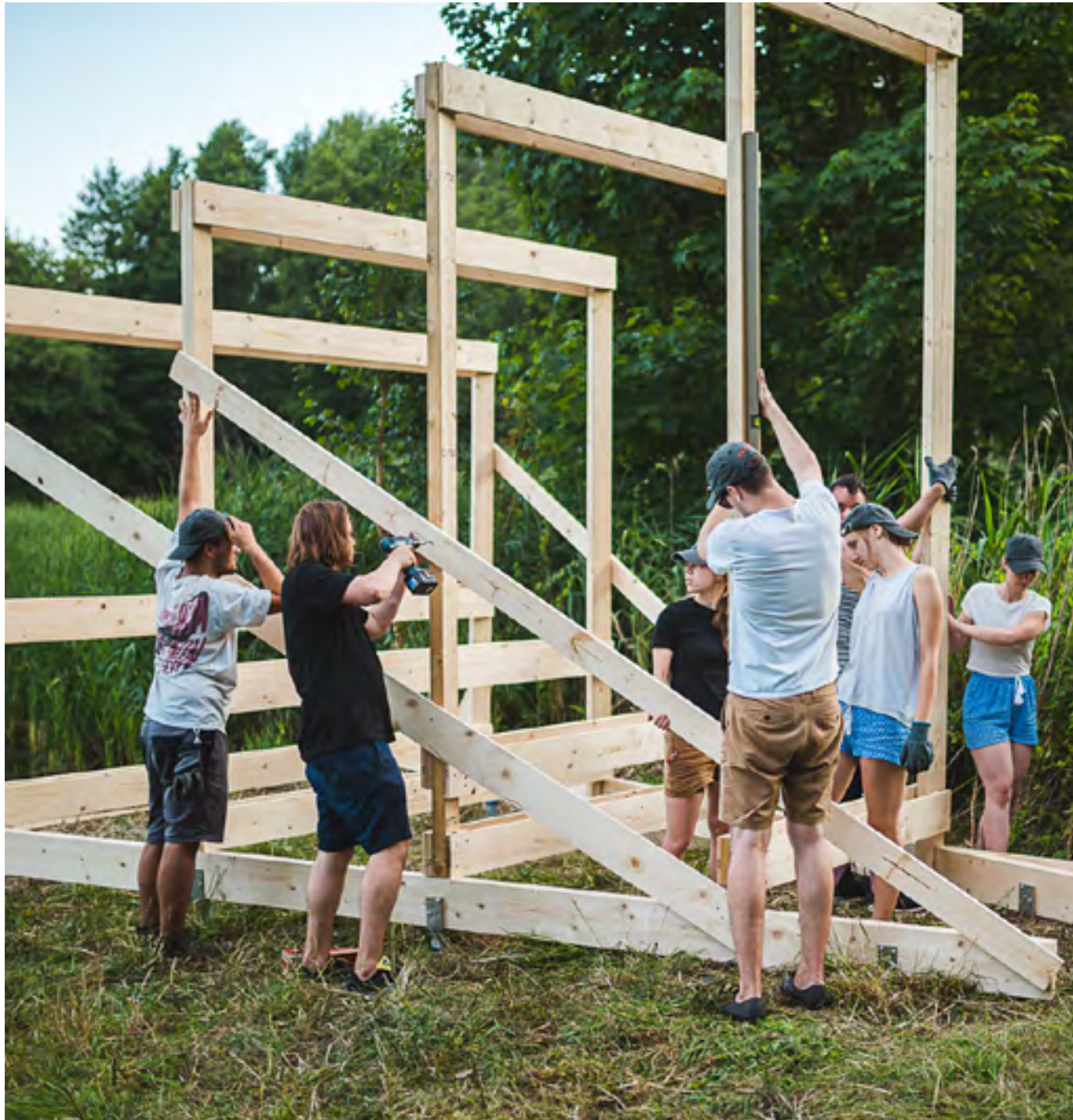
Constructing working at the location site
