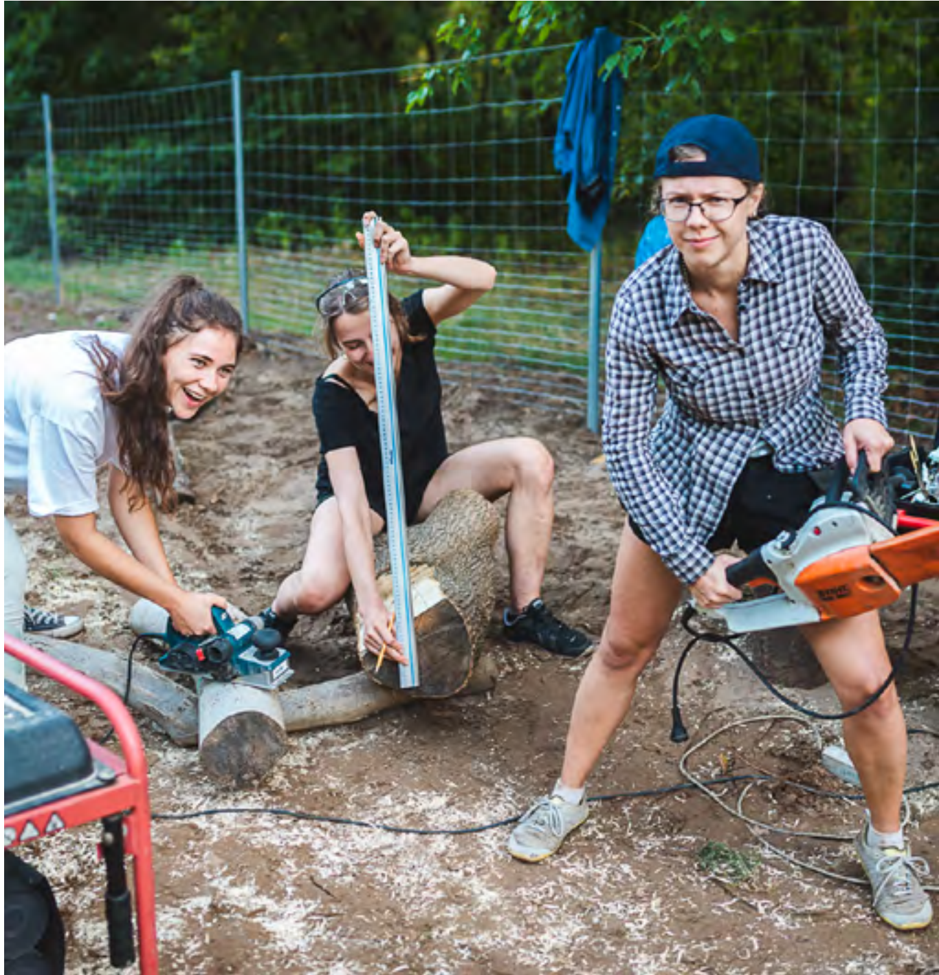
Constructing working at the location site
