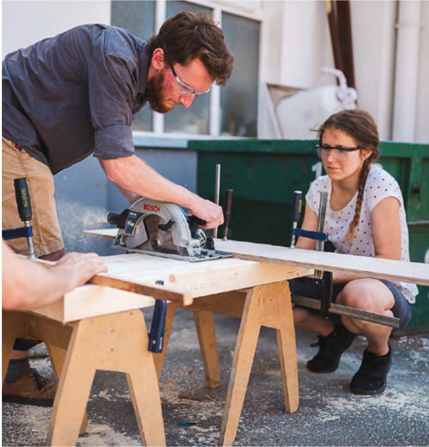
Constructing working at the location site
