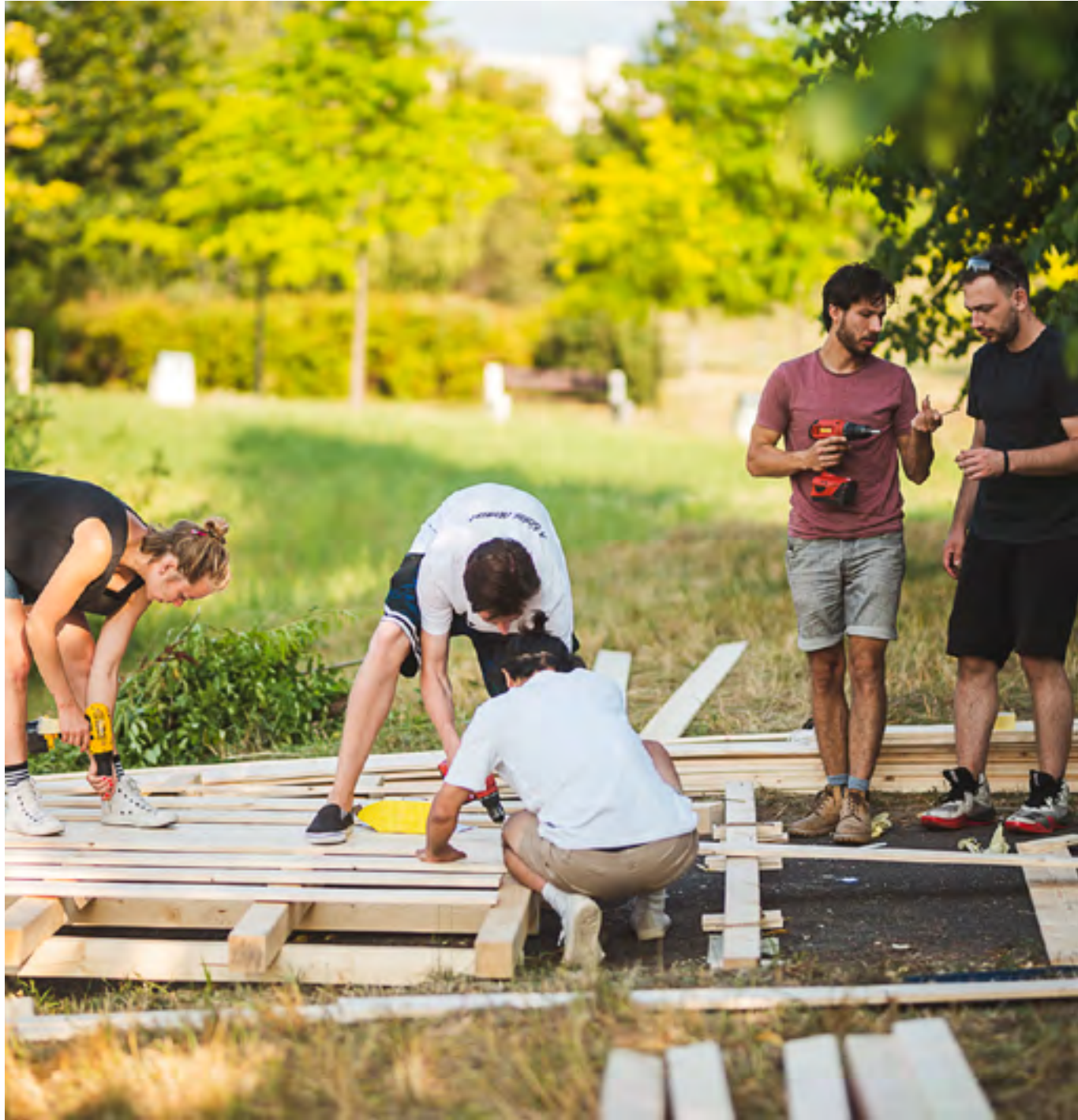
Constructing working at the location site
